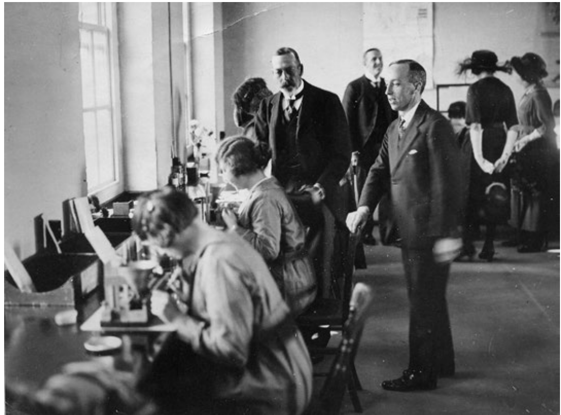
The new building on Huntingdon Road was completed in October 1921, and officially opened on 14 October by HM King George V and Queen Mary
